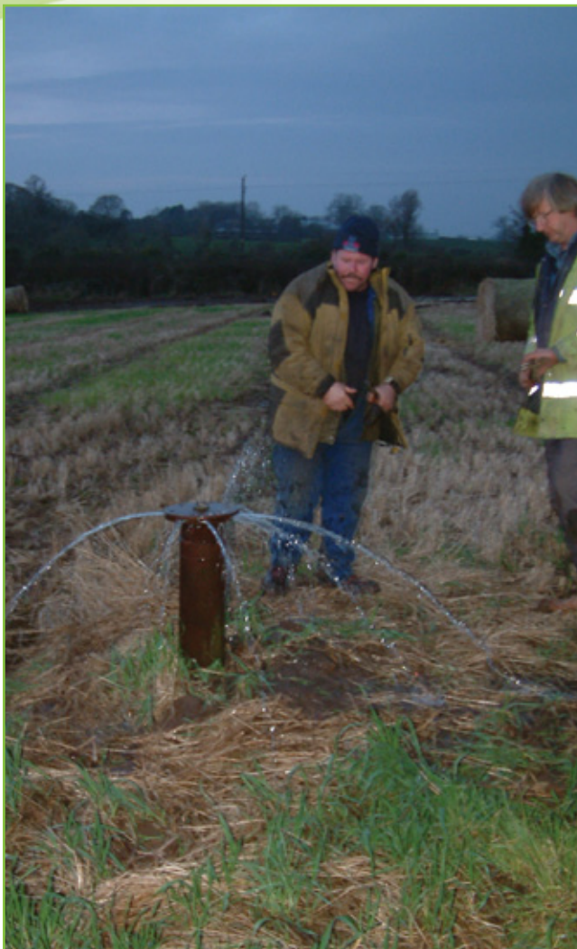
PICTURE ABOVE: Capping an artesian borehole
